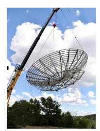
The dish lifted in the air by a crane and rotated to the birdbath
